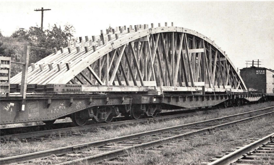
Oversize shipments like this hundred foot laminated wood roof truss receive special attention.
