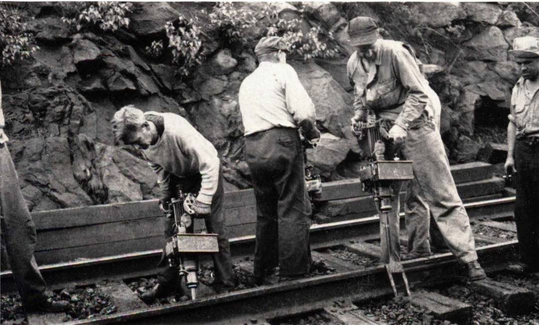
Modern machine methods are used by Maintenance workers to speed track repairs.
