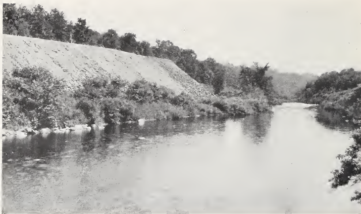
a. View looking down the Shepaug River from below the site of the proposed dam. Part of the dump from the tunnel excavation is shown at the left.
