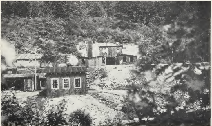
b. View looking into entrance of tunnel from across the Shepaug River, along the line of the proposed dam.
